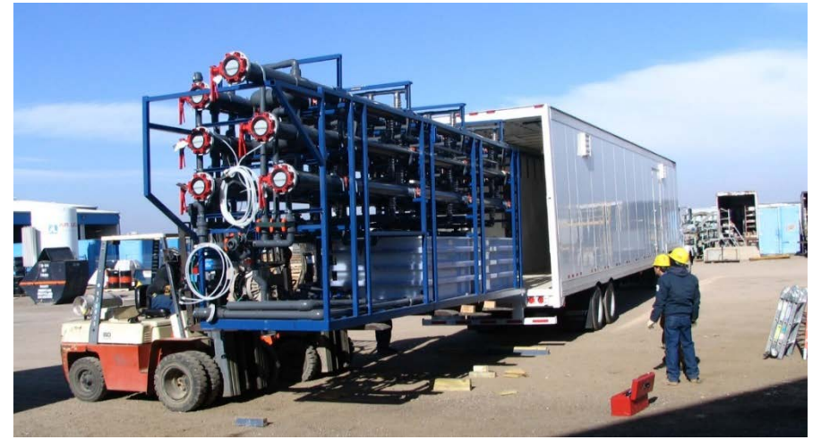
System fabricated in three 48 ft trailers off site in Colorado
